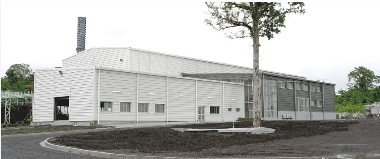
Fiaga 20MW Diesel Generation Station
