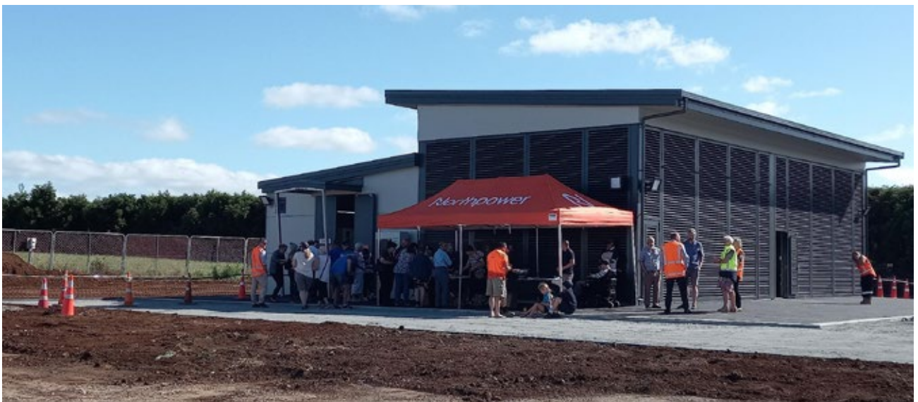
The new Maunu substation is a $6.6 million investment supporting growth in the area (up to 5,000 homes and businesses) and providing an alternate supply to Whangārei hospital and CBD.
